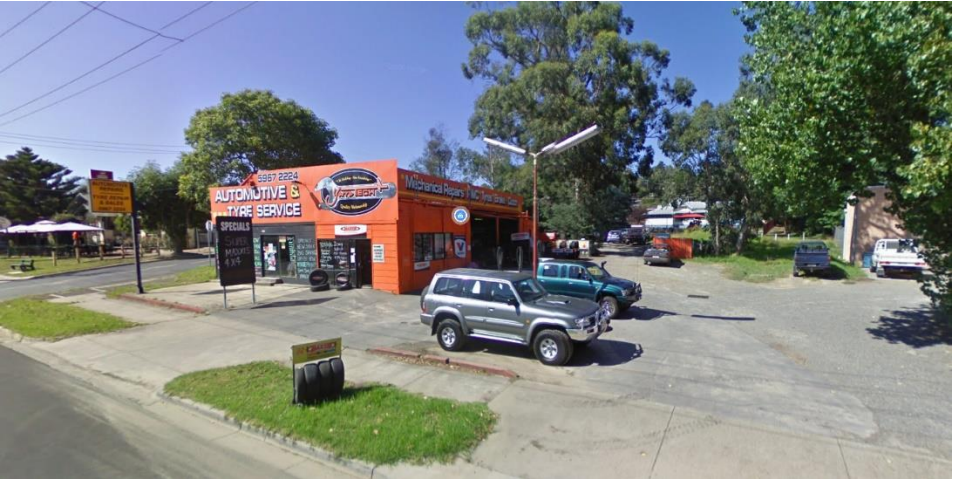
Figure 2 - Existing building on subject site viewed from Warburton Highway
